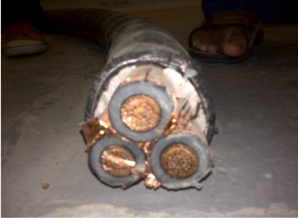
Figure 14: The High voltage side cable cut and ready to be connected. The cables are thin because the voltage is high but the current is low.
