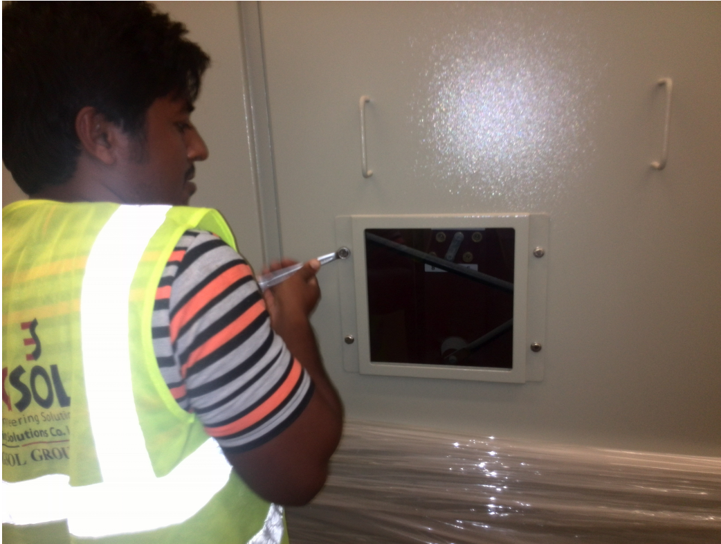
Figure 16: The cavity for changing the transformer taps by using the wrench tool.
