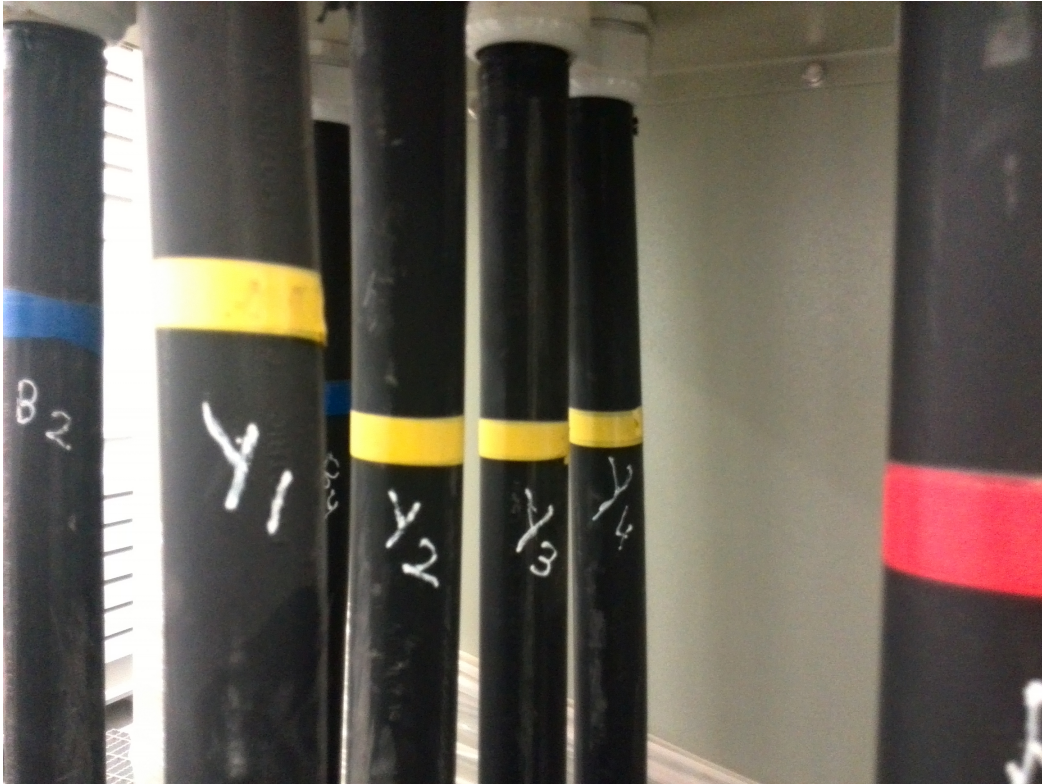
Figure 10: The Red phase wires on the low voltage side of the transformer.
