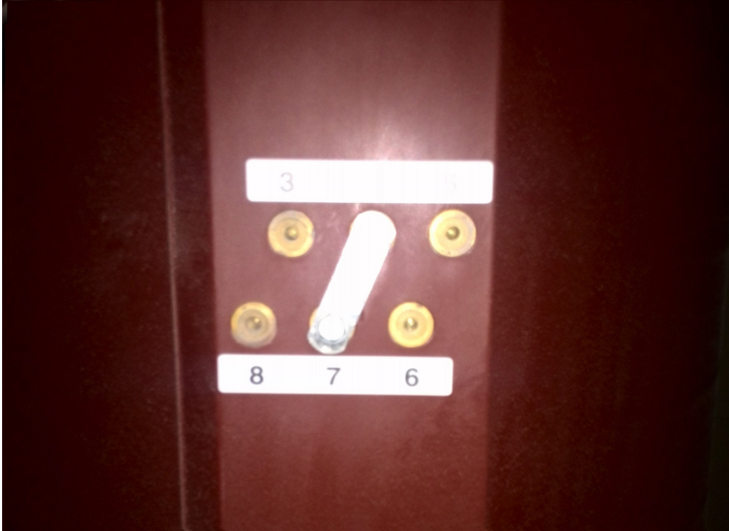
Figure 18: The transformer taps with numbers clearly shown.
