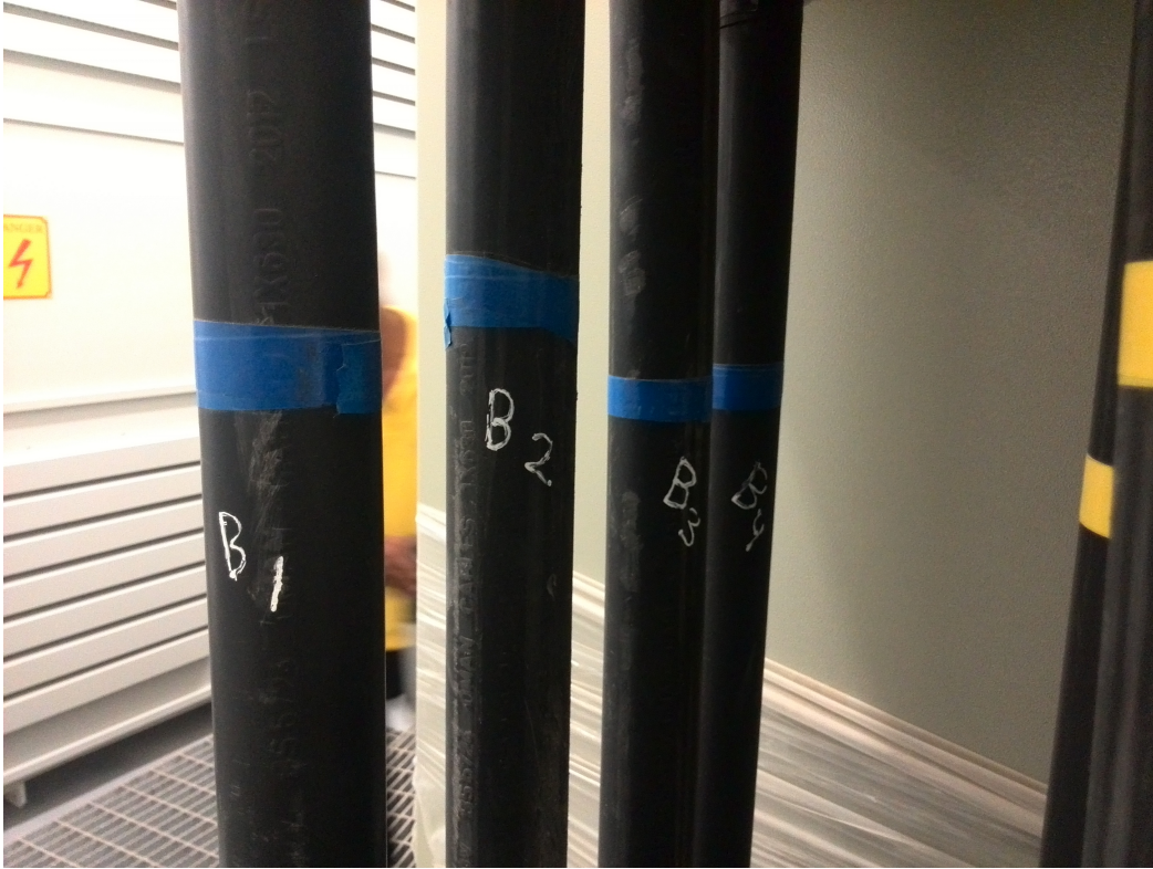
Figure 12: The Blue phase wires on the low voltage side of the transformer.
