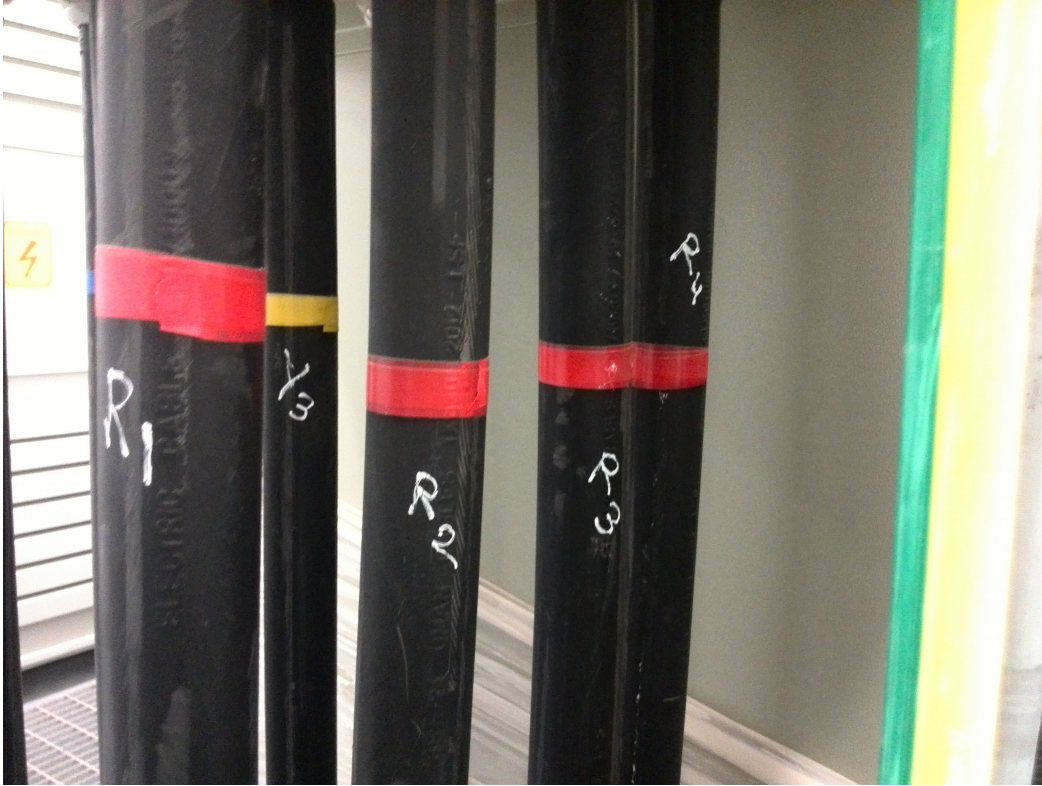
Figure 10: The Red phase wires on the low voltage side of the transformer.
