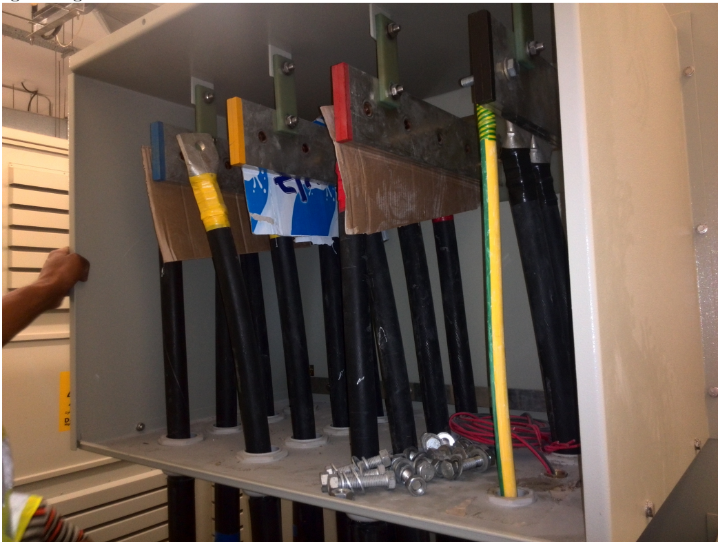
Figure 14: The High voltage side cable cut and ready to be connected. The cables are thin because the voltage is high but the current is low.
