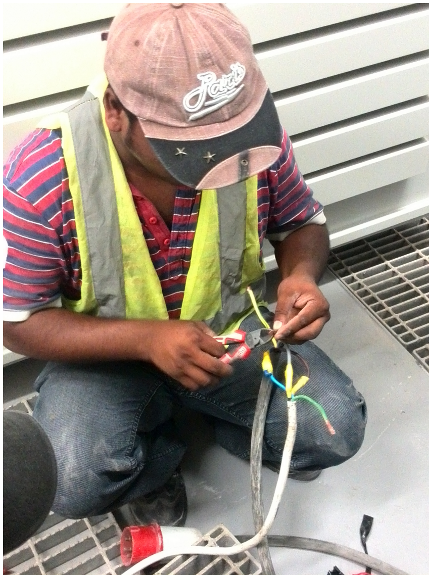
Figure 32: The wires are being cut for the three phase supply to the high voltage side.
