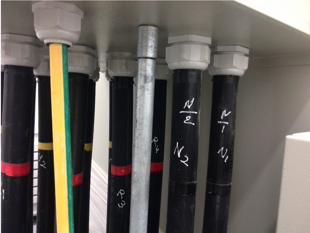
Figure 12: The Blue phase wires on the low voltage side of the transformer.
